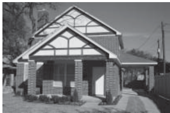
The new home at 2314 W. Rosedale South is now complete and fits nicely in the neighborhood.
