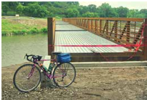
The span of the pedestrian/bike bridge has been completed. This photo was shot before the surface was laid on the bridge.
