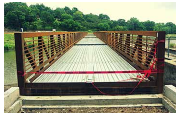
The span of the pedestrian/bike bridge has been completed. This photo was shot before the surface was laid on the bridge.
