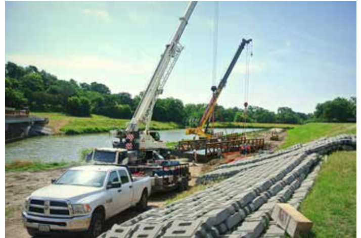
Large cranes were used to lift the bridge spans into place atop the concrete piers.
