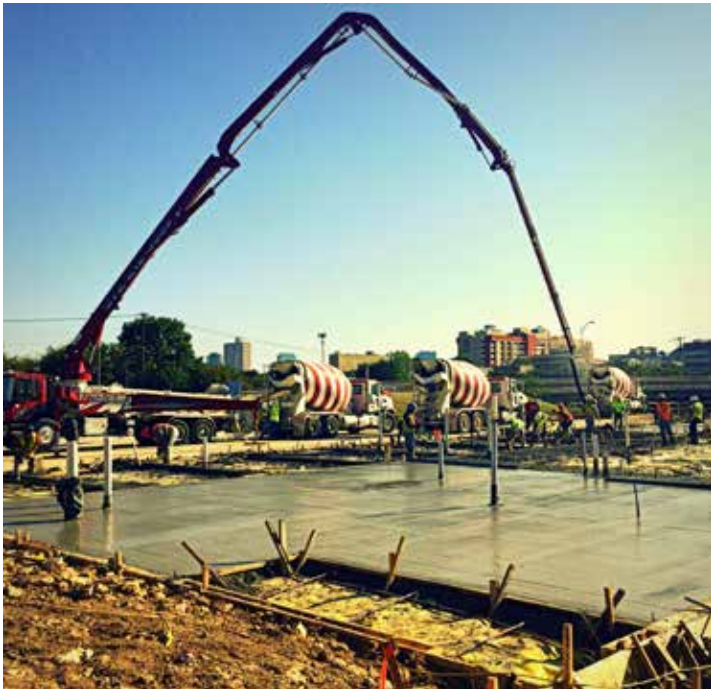
Pouring the foundations for Magnolia on Rosedale, a 35-unit residential complex at Jerome and Rosedale streets
