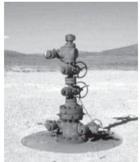
A gas well after drilling is complete.
