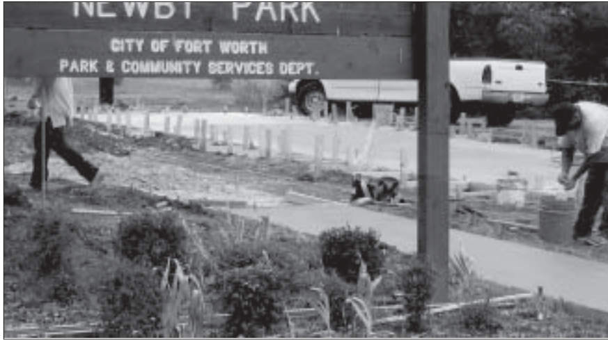
The pavilion's slab has been poured.
