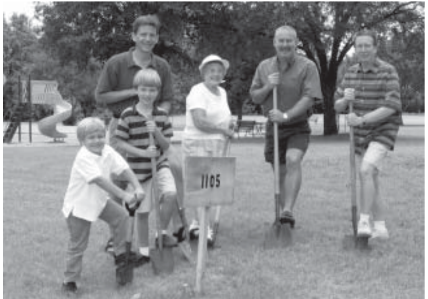
Unofficial ground-breaking at the site of the Newby Park Pavilion. Pictured are a few of the pavilion committee members: Jim Bradbury and sons, Sam and Jack, Patsy Slocum, John Key, and Martin Herring.
