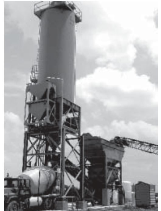
An view of a typical concrete batch plant.
